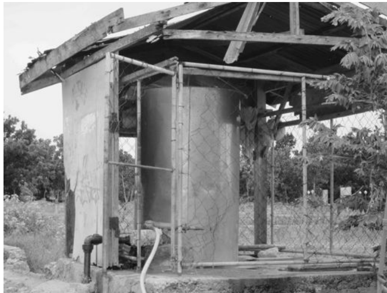
Figure 3. A water tank in Cordova. (Photo by the author.)
